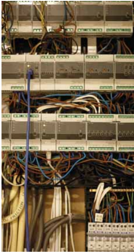
figures 3.18a Preparation of the prototype, extra measurement modules are installed in the Niko Home Control system.
