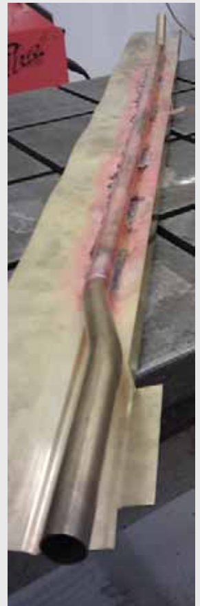
Figure 48: Soldering radiator panels and tubes
